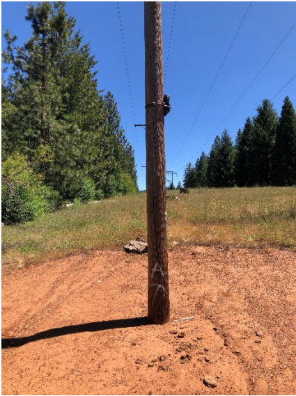
LT-1 Looking Northeast
