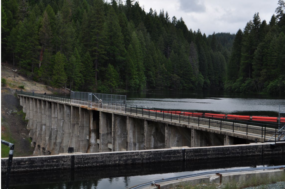
Key View 5. View from near the existing spillway structure looking north toward the dam and reservoir.
