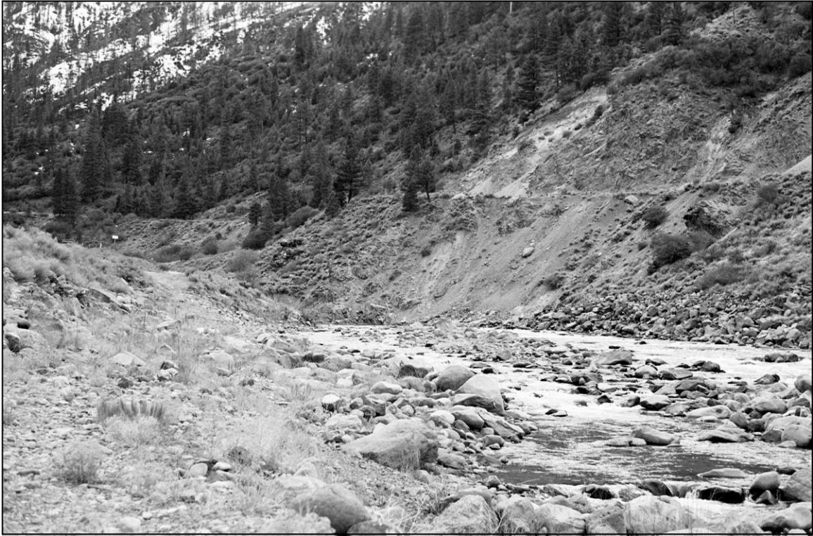
View of the project construction area looking southwest (upstream) toward old Highway 40.
