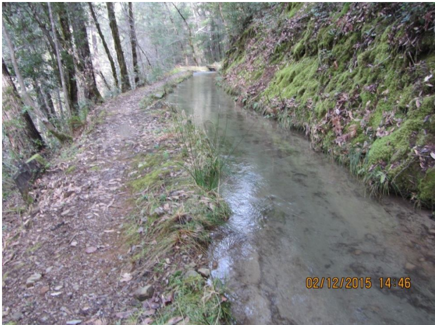
Image 14- shows point 8, an approximately 150-foot section of the channel downstream of Point 7, where the low berm and full ditch likely creates a high potential for berm or slope failure, erosion, and sediment transport downslope. I observed concrete blocks at various locations along the outboard edge of the berm throughout this segment, likely to rebuild or reinforce berm sections. (Photo 8486)
