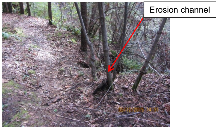
Image 6- shows the erosion channel downslope of Point 3.
