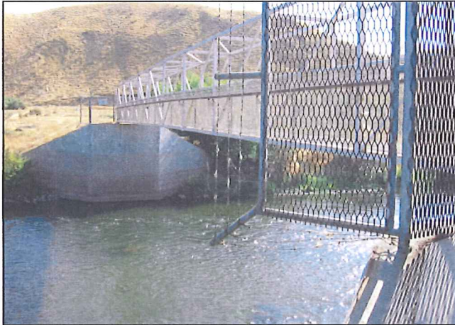
Photo a: Kern River, First Point of Measurement (First Point) at controlled channel cross section and gaging station. Recorded flow rate of 508 cfs on 9/30/09.
