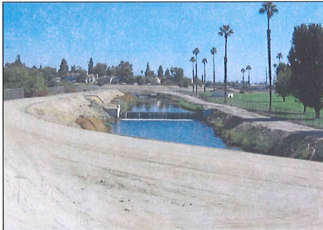
Photo i: Carrier Canal just downstream of Four Weirs diversion station and west of Manor St.
