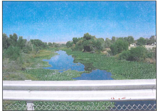
Photo d: Kern River at Manor Street looking upstream. River ponds behind gates at Riverview Park (Photo 10h) creating stagnant flow condition upstream of Manor Street. Note abundant growth of water primrose.
