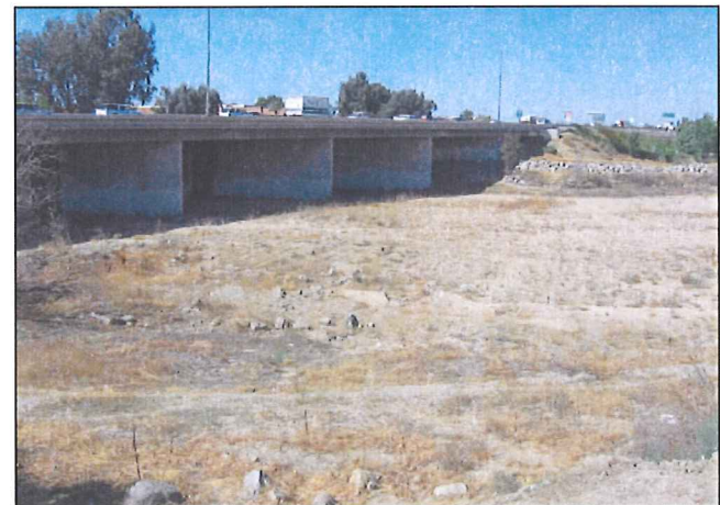
Photo l: Kern River upstream of Hwy 99 crossing. Dry channel bed, sand and gravel deposited upstream of crossing.
