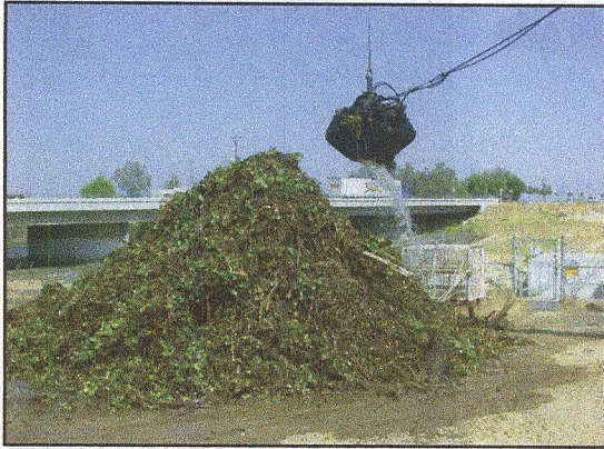
Crane removing debris from head of River Canal
