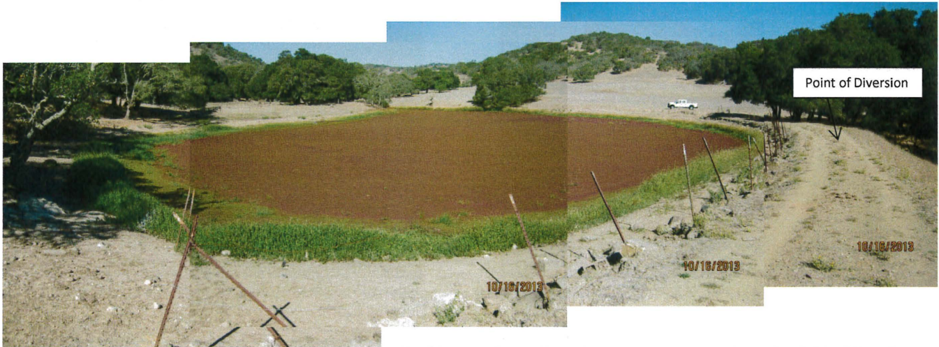
Figure 30: Reservoir as seen from the southeast corner looking north. Earthen dam runs northeast along the right of the photo.
