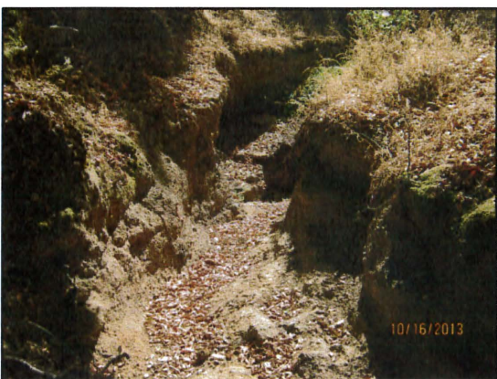
Figure 62: Defined spillway channel looking south.
