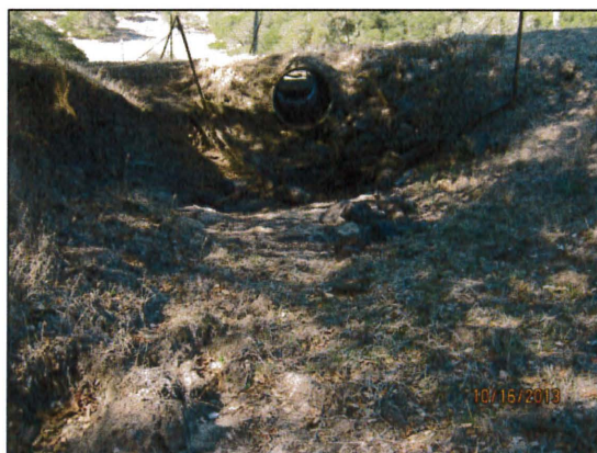
Figure 51: The spillway outlet as seen from the downstream channel.
