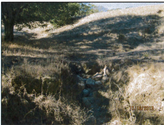
Figure 86: Unnamed Stream at the base of the earthen dam.
