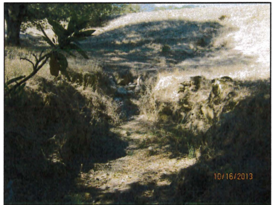
Figure 85: Unnamed Stream looking northwest towards the base of the earthen dam.
