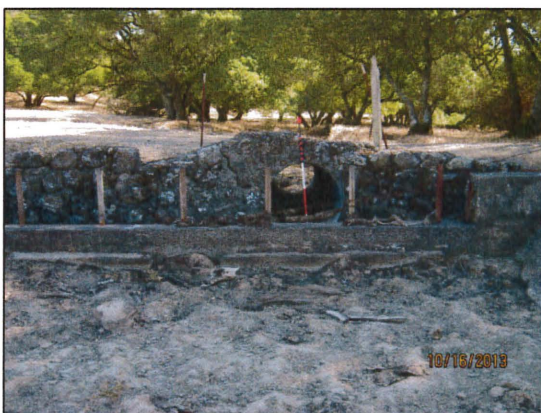
Figure 50: Reservoir spillway and cement wall.
