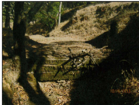
Figure 23: Unnamed Stream as seen looking northwest, upstream, at the flashboard dam.
