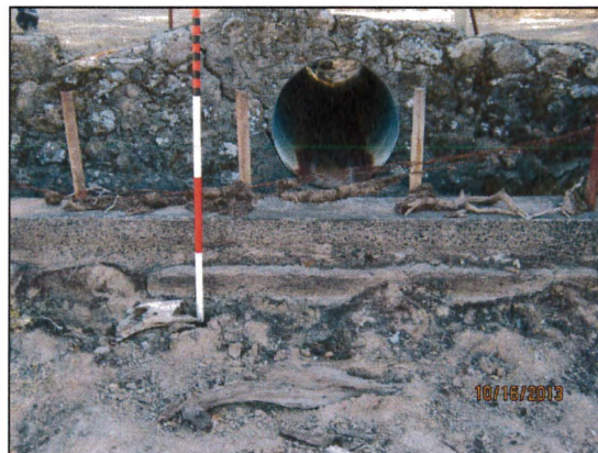
Figure 49: Survey rod in front of the cement wall for perspective.
