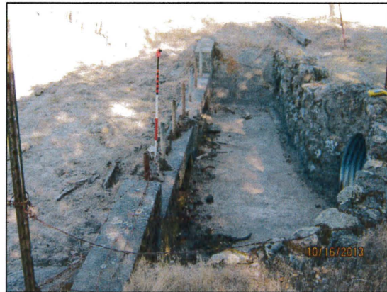
Figure 47: Cemented area between the cement wall and the spillway.
