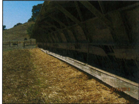
Figure 89: Close up of one of the facilities. Hay was scattered around the facility and stored inside as well.
