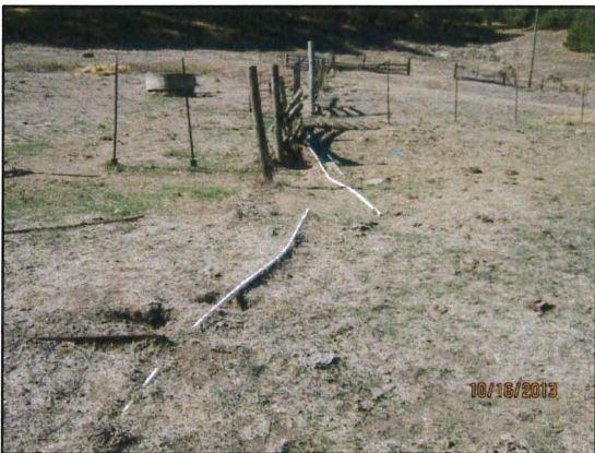
Figure 90: PVC piping running along the fence line as seen looking east.
