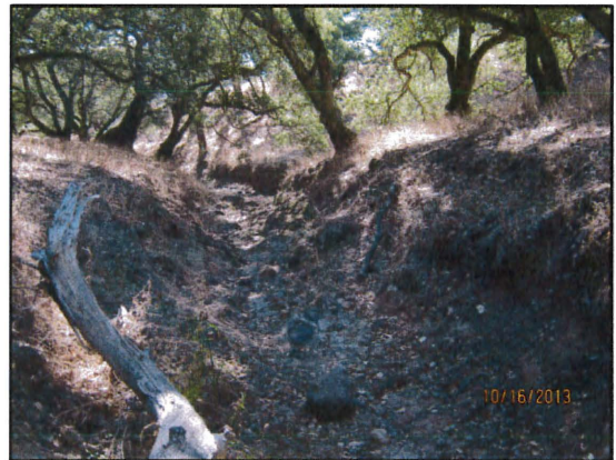
Figure 61: Defined spillway channel looking south.
