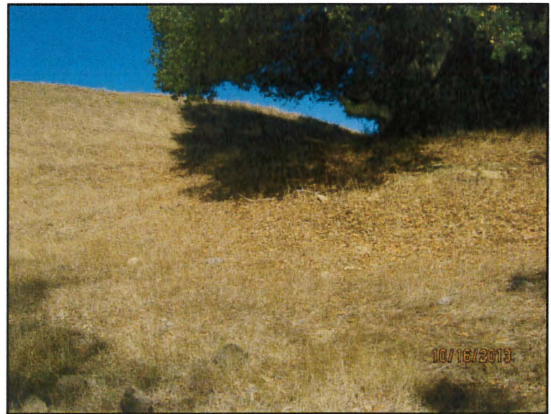
Figure 87: Earthen dam as seen looking north from the Unnamed Stream.
