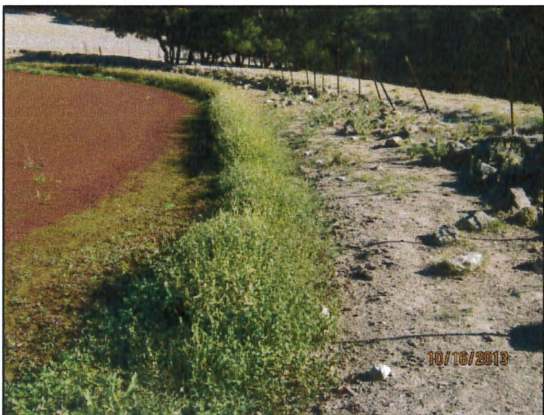
Figure 36: Southern point of the reservoir looking northeast along the dam.
