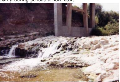
The Highway 1 Bridge apron presents a low flow fish passage impediment on lower Salsipuedes Creek.
