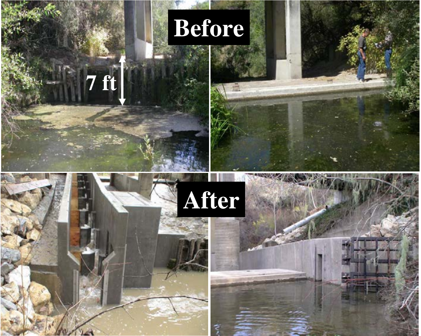
Figure 10: Fish passage and habitat restoration in the fall of 2008 at Rancho San Julian on El Jaro Creek.
