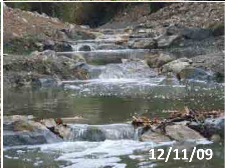
Figure 12: Fish passage and habitat restoration in the fall of 2009 at Cross Creek Ranch on El Jaro Creek, a tributary of Salsipuedes Creek and the Santa Ynez River.
