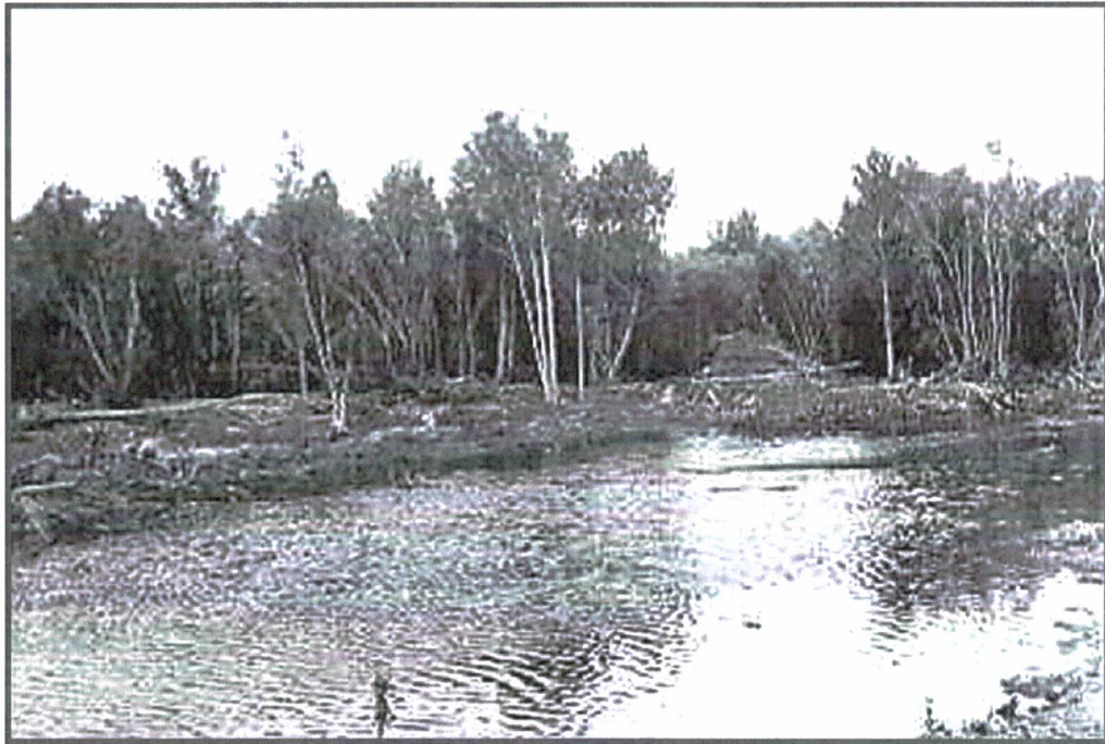
Fig. 12. Flood control operations between the Alisal Bridge and the Santa Rosa ranch conducted by the County of Santa Barbara, Public Works Department, November 1944. Note mature riparian vegetation along the lower mainstem of the Santa Ynez River, in the vicinity of Hollister's ranch. Mark H. Capelli Southern California Steelhead Watershed Archive, UCSB Donald C. Davidson Library.
