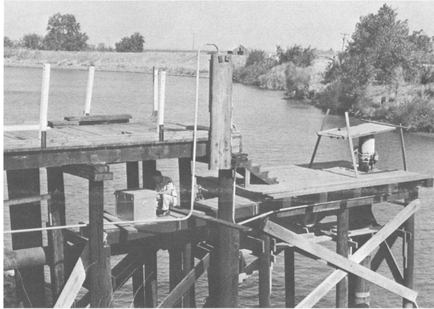
FIGURE 9. Monitor housed on an irrigation pump platform, San Joaquin River near Bowman Road, fall 1965. Photograph by John A. Shaver.
