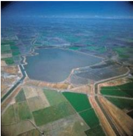
Aerial view of Clifton Court Forebay
