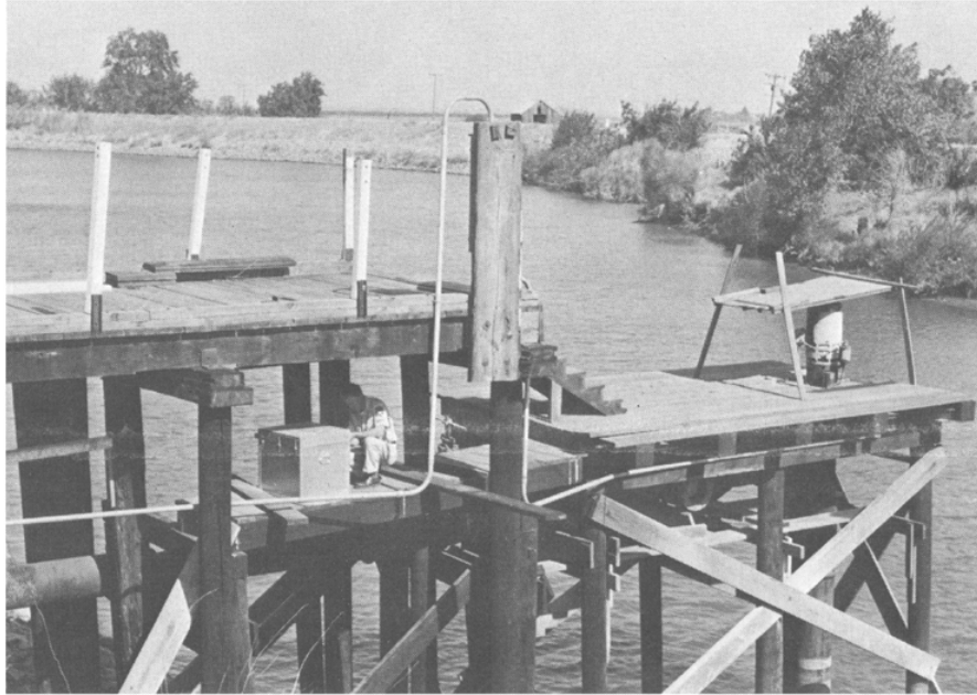
FIGURE 9. Monitor housed on an irrigation pump platform, San Joaquin River near Bowman Road, fall 1965. Photograph by John A. Shaver.
