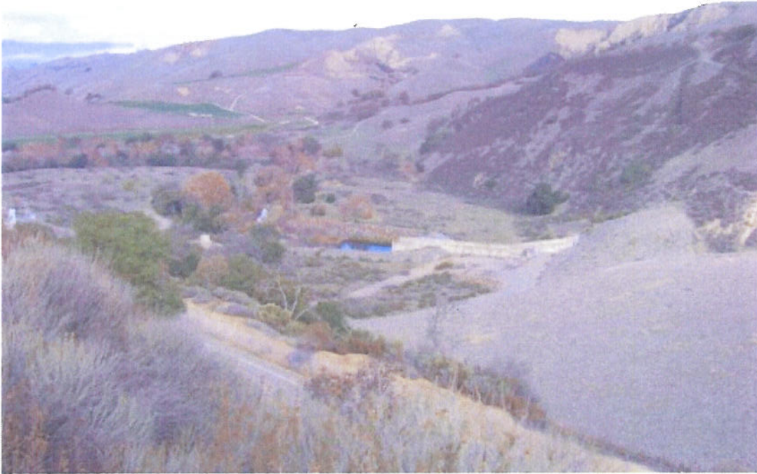
Arroyo Valle Channel – Below Lake Del Valle Dam (POD #1)
