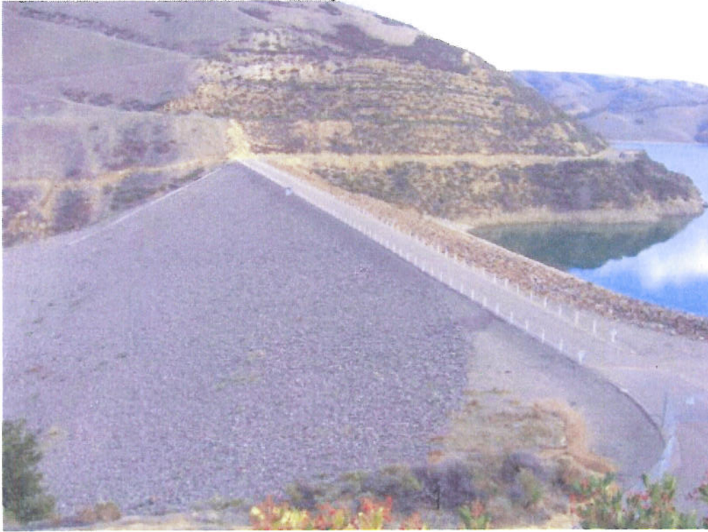
Point of Diversion #1 (Lake Del Valle Dam)
