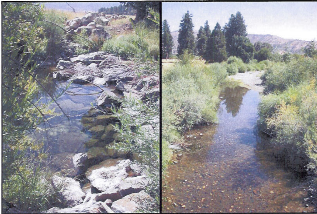
Photo 1. Photographs of lower French Creek showing one of the vortex weirs at Diversion No. 48 (left) and the conditions of the stream channel upstream (right). Photos are courtesy of the Scott River Water Trust.
