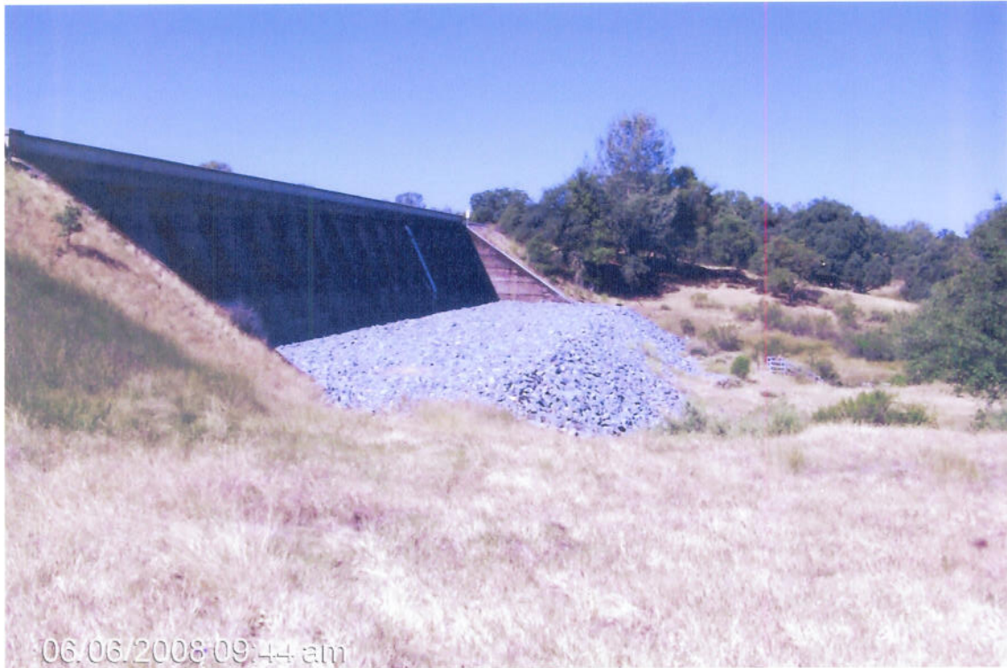
NORTH SPILLWAY AT PARDEE LOOKING WEST
