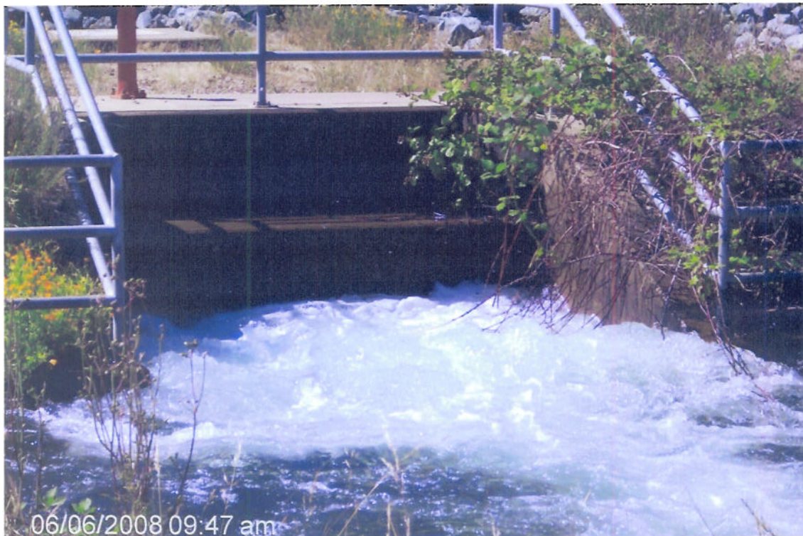
WATER BEING RELEASED OUT OF NORTH SPILLWAY OUTLET
