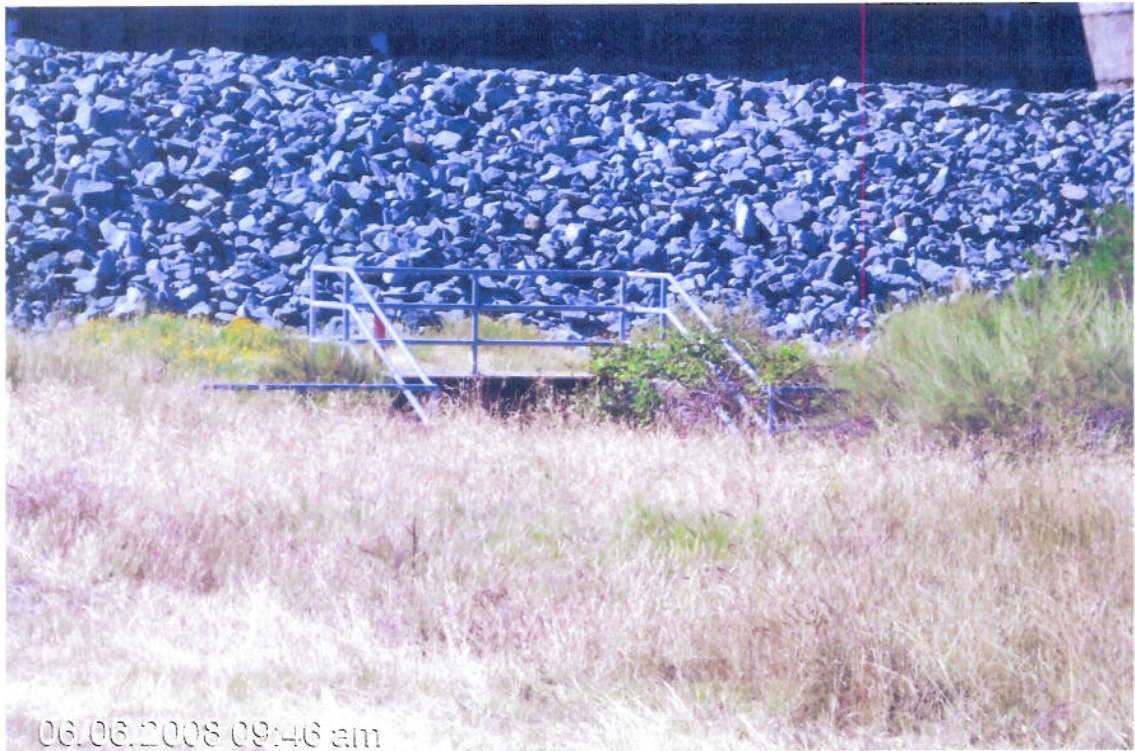
NORTH SPILLWAY OUTLET AT PARDEE
