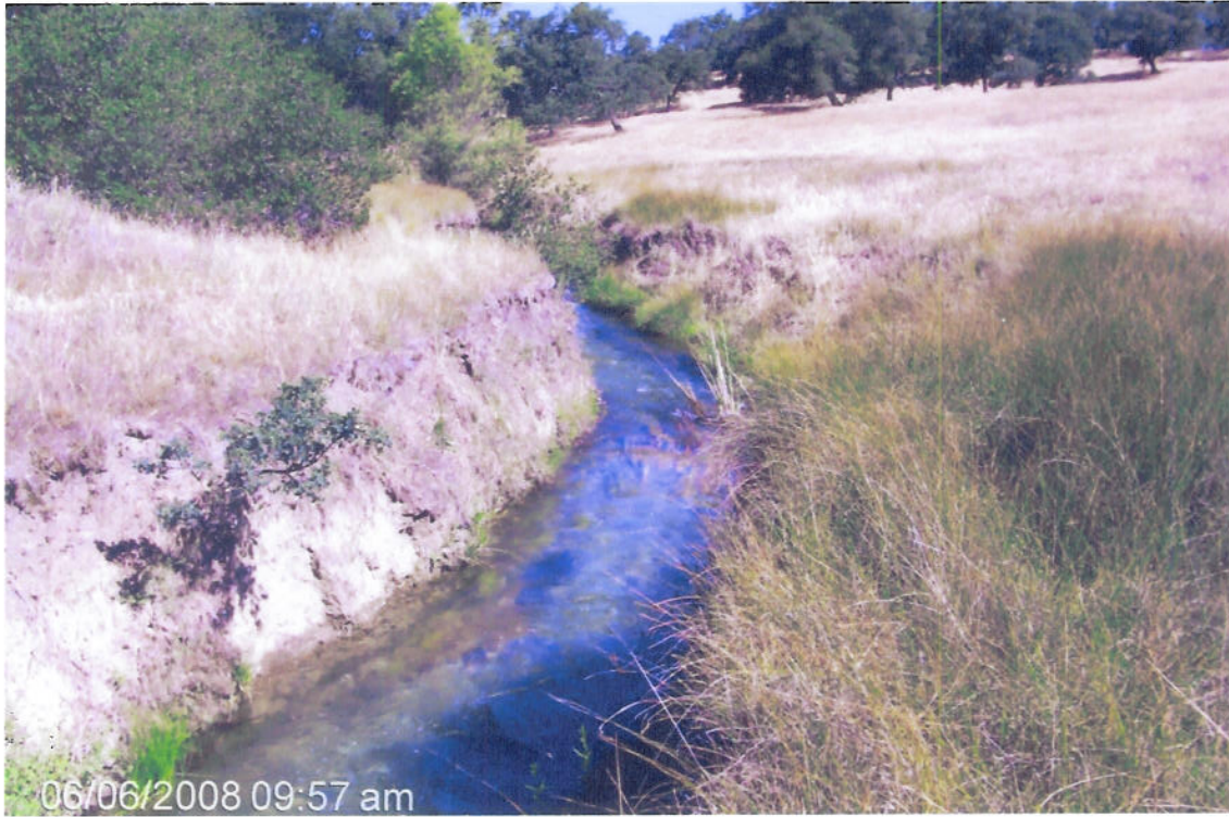
200' DOWNSTREAM OF NORTH SPILLWAY OUTLET LOOKING DOWNSTREAM
