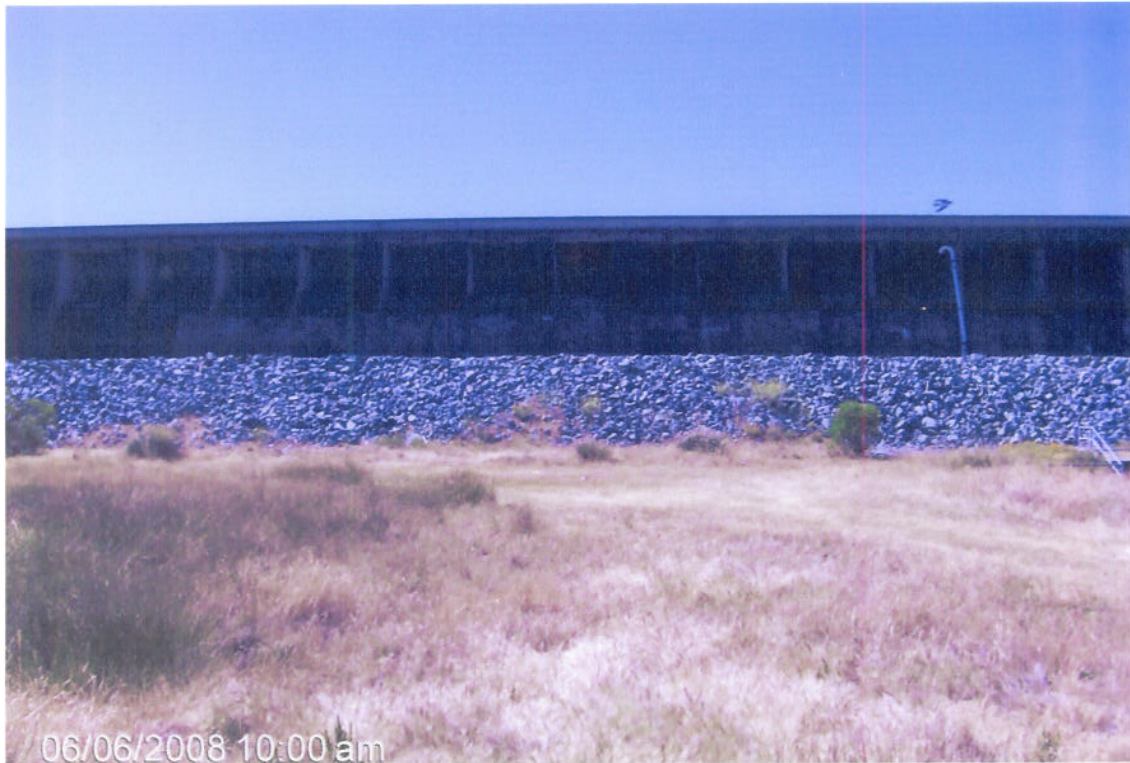
NORTH SPILLWAY AT PARDEE LOOKING SOUTH
