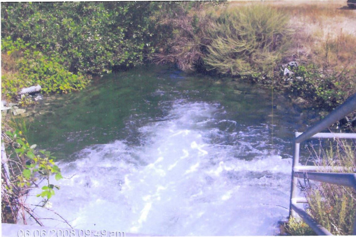
JUST DOWNSTREAM OF NORTH SPILLWAY OUTLET
