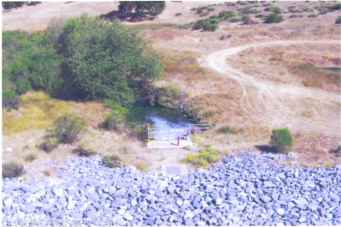
LOOKING NORTH FROM ON TOP OF NORTH SPILLWAY AT OUTLET
