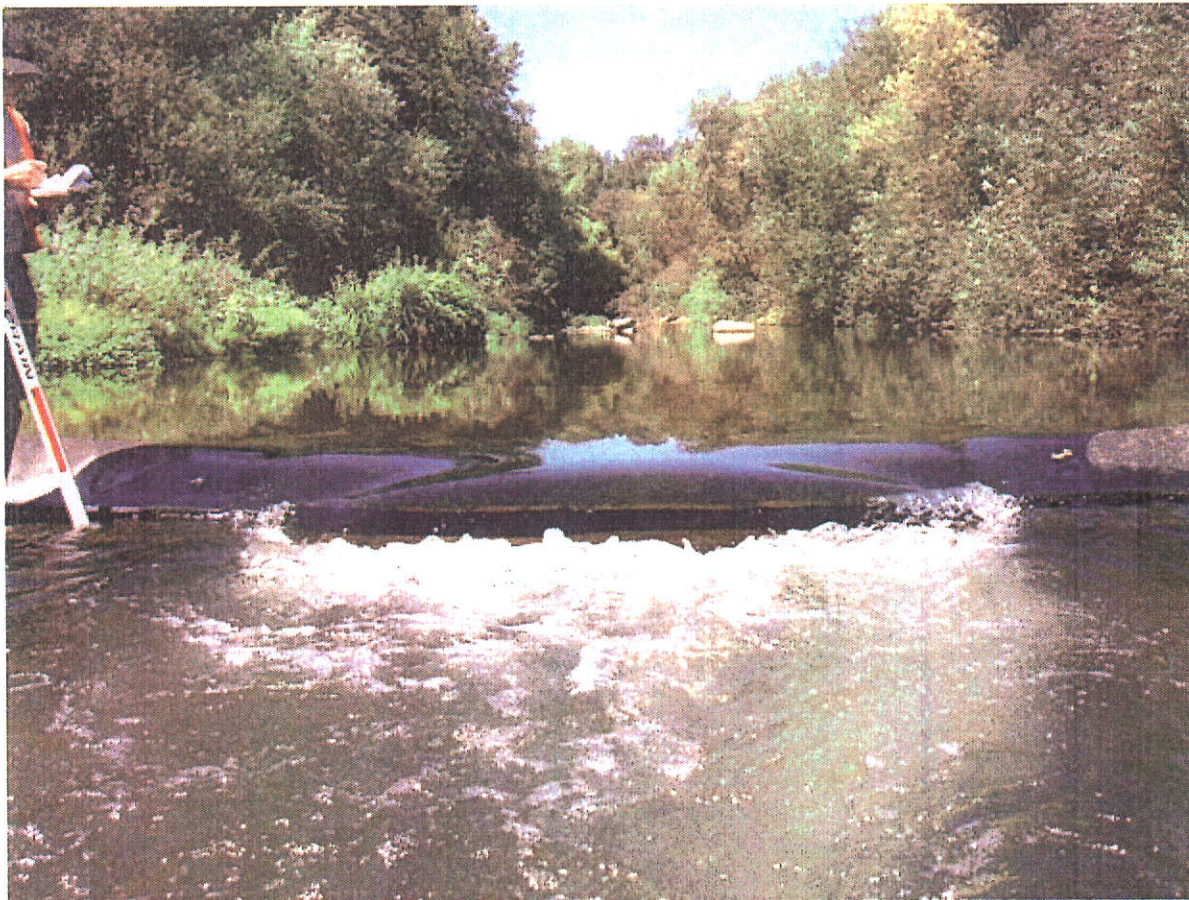
Felton Diversion Facility on San Lorenzo River Looking upstream during low flow.
