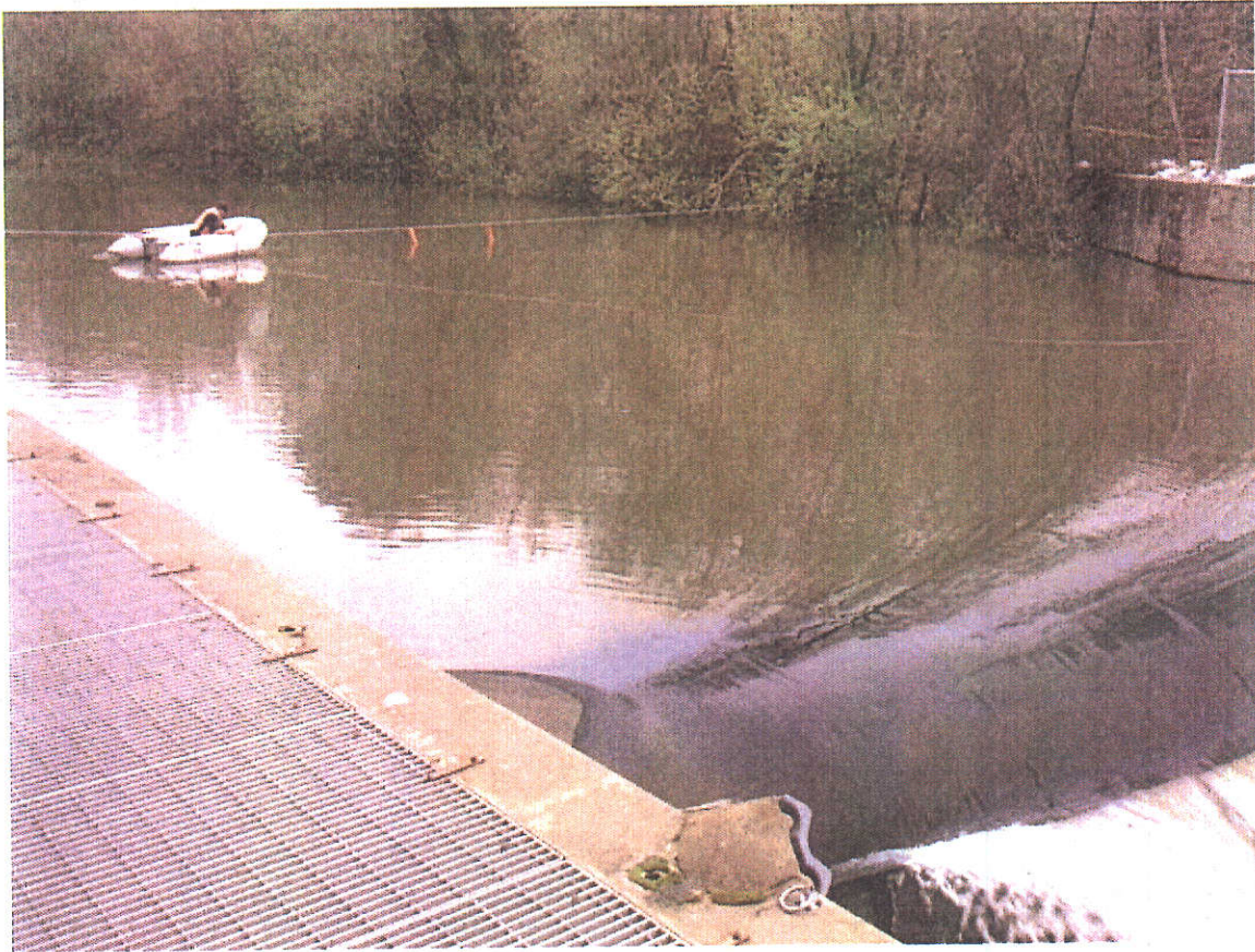
Felton Diversion Facility on San Lorenzo River Looking upstream during high flow.
