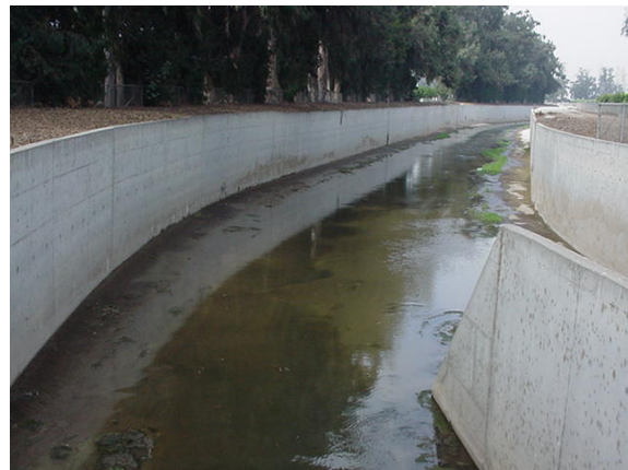
Looking northwest in concrete lined channel
