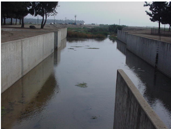
Looking towards natural unlined channel (east)
