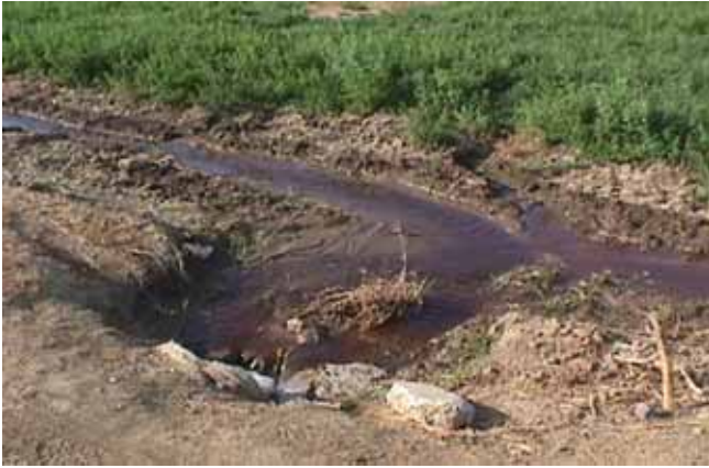
Figure 34: Del Puerto Creek 10 meters upstream of Vineyard Road
