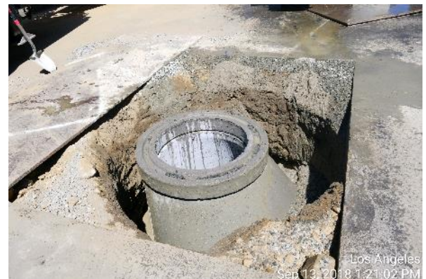
Top of Drywell
