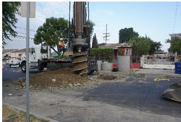
Drilling of Drywell Shaft
