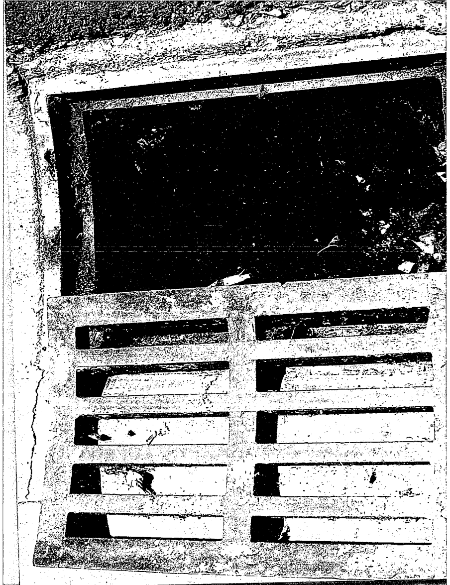
Storm Water Drain
