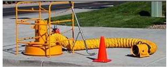
Manhole guard, ring blower/hose
