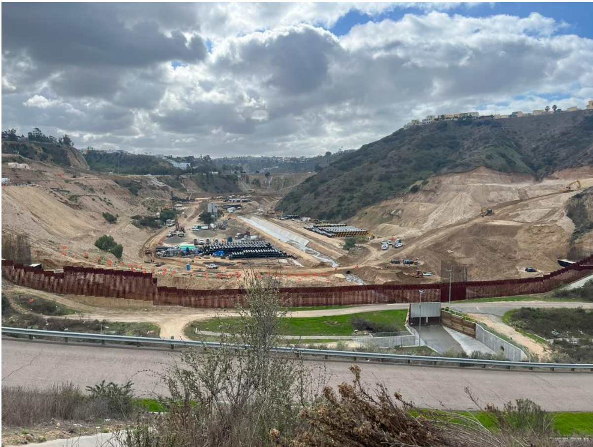
Figure 13: Mexican construction project in Matadero Canyon. (MC 01/10/2024)
