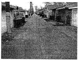
Figure 10: Permeable Pavers and Permeable Concrete Chicago Alleys (Source: Abby Hall, US EPA)
