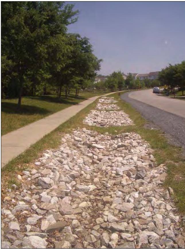
This swale can capture runoff from the adjacent road. Some swales, like this one, are lined with rocks, while others are lined with vegetation and other media like mulches.
