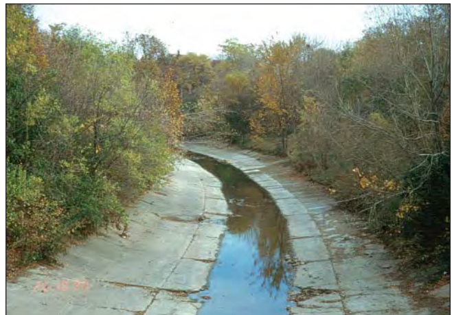
Conventional grey infrastructure is efficient at carrying large volumes of stormwater away from our built landscapes, but not without contributing to water pollution and streambank erosion problems.
