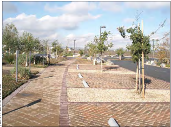
Parking spots with permeable pavement.
