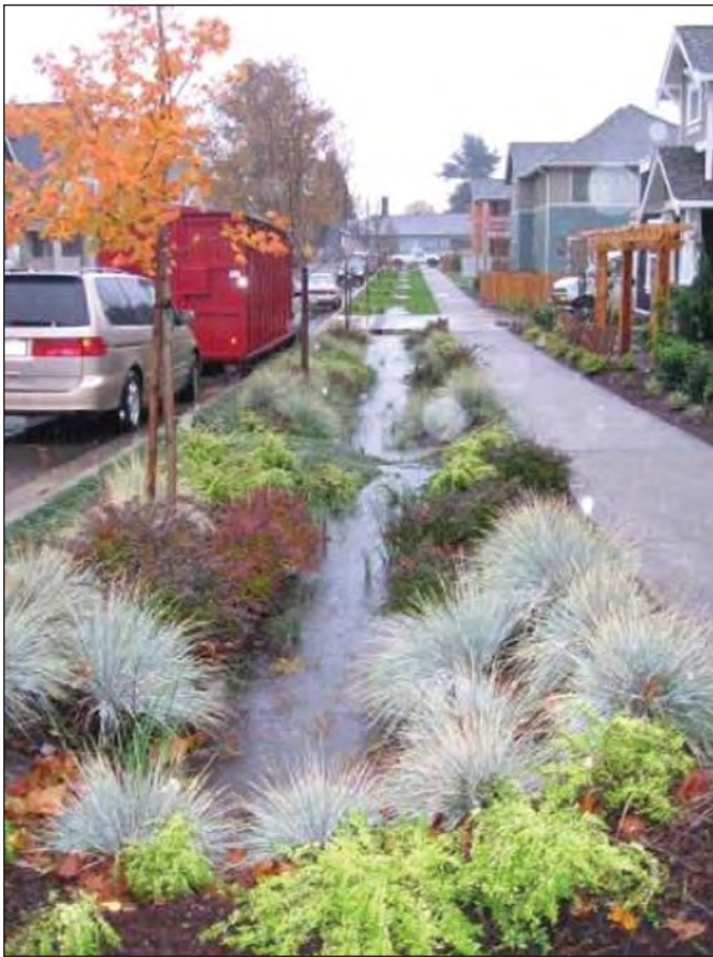
Natural vegetation helps catch and filter runoff in this example of green infrastructure at work.
