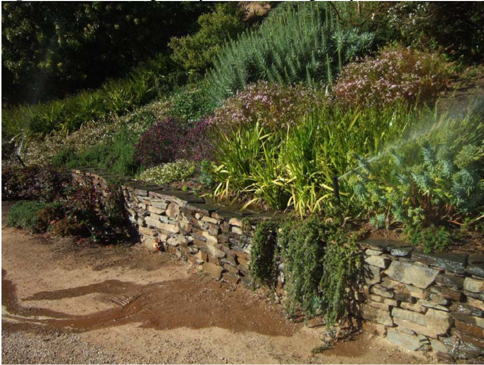
Figure 2-3. Private irrigation system contributing to dry-weather runoff
