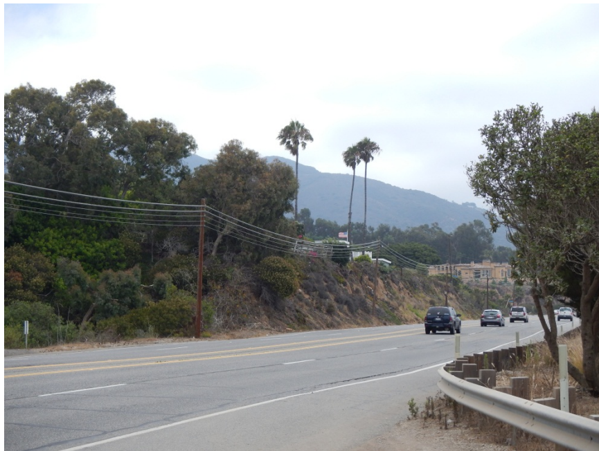
Figure 7-8. Directly Above Broad Beach Area
