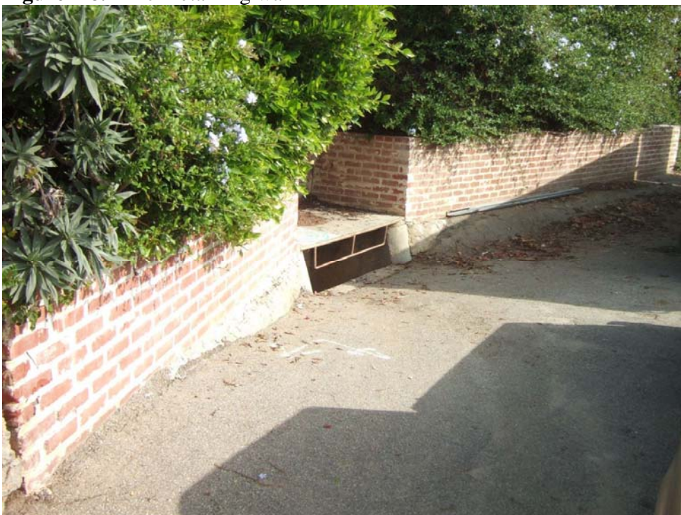
Figure 2-8. Brick retaining wall
