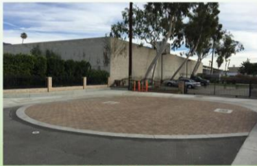
SUBSURFACE INFILTRATION BASIN
