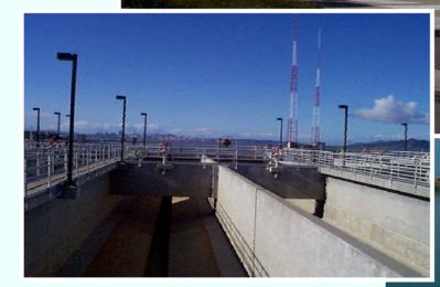
Design Flow: 100 MGD Storage: 3 MG Treatment: Screening, Sedimentation, Chlorination, Dechlorination
